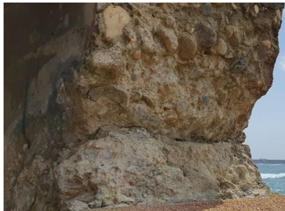
Large volume loss and shrinkage / thermal movement
