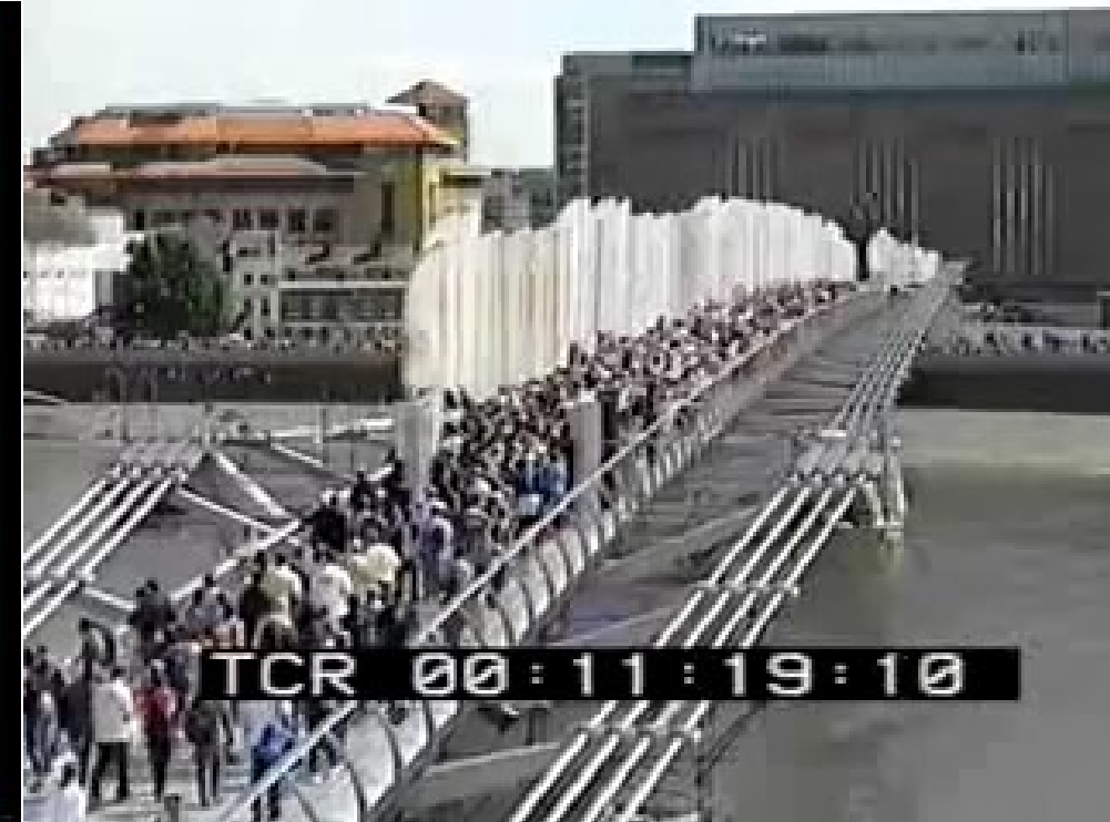
Millennium Bridge, 2020 Lateral frequency modes
