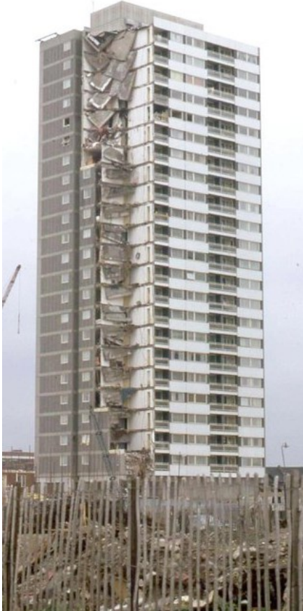
Ronan Point, 1968 Disproportionate collapse
