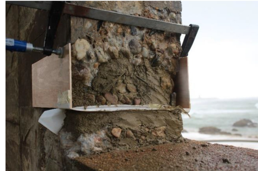
Mold, silicon paper and mortar filling
