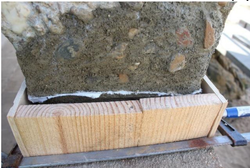
Mold, silicon paper and mortar filling
