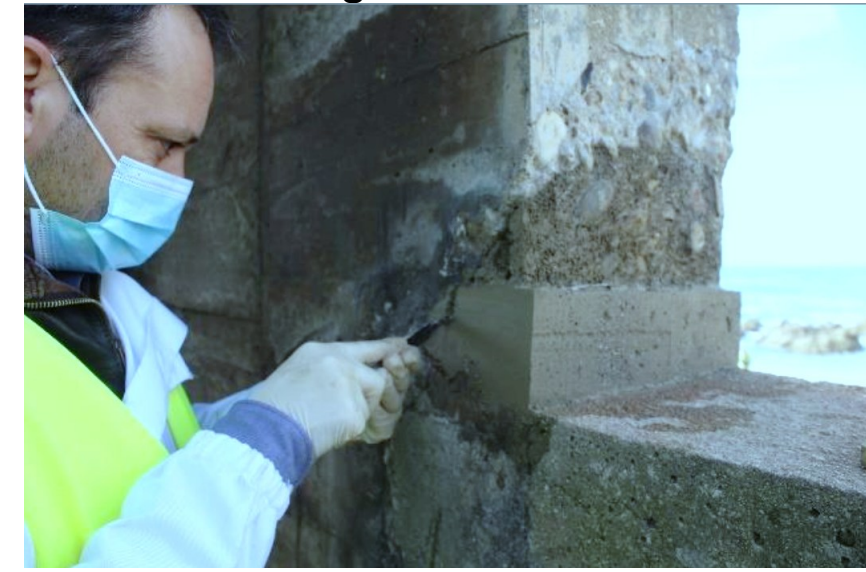
Mold, silicon paper and mortar filling
