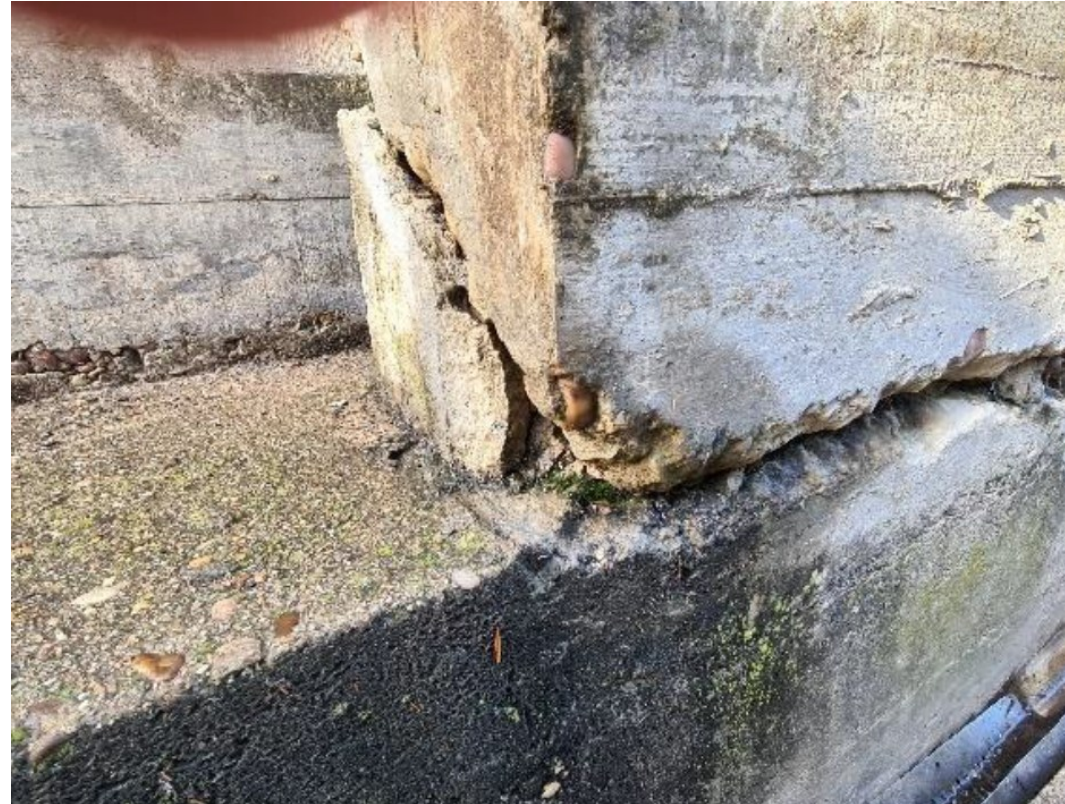
Displaced fragment, volume loss and biological colonization
