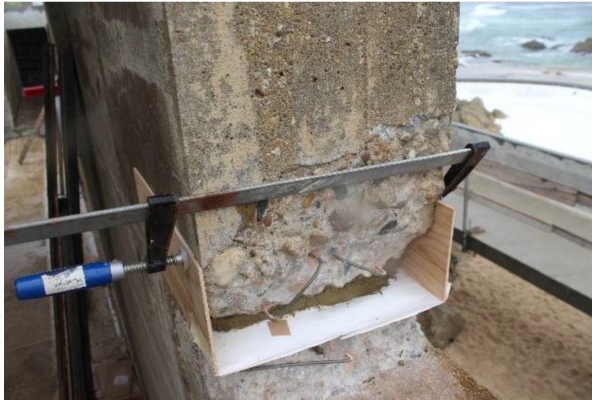
Mold, silicon paper and mortar filling
